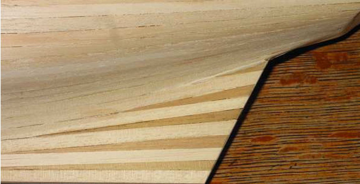
Photo 1: Triangle-shaped filler planks – darkened in the photo for contrast.
